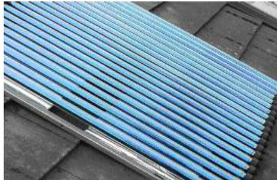
**Fig.5. Plain Tube collector**
